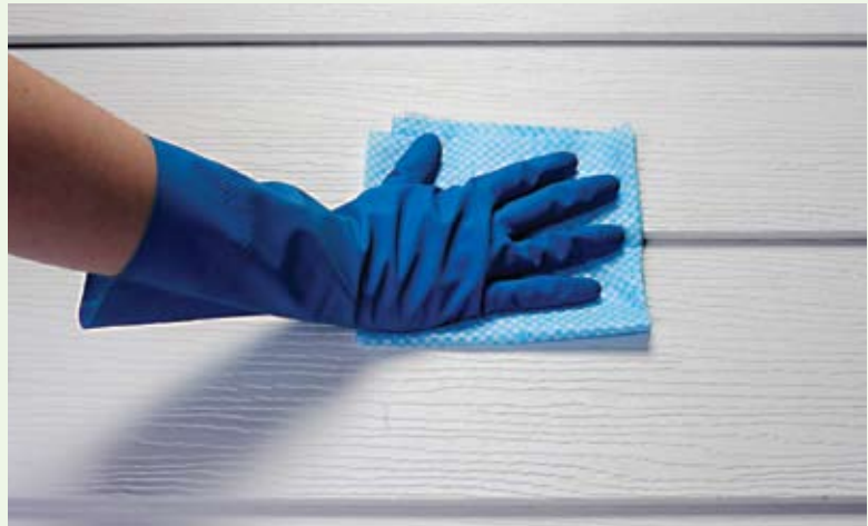
...but a quick wipe down will keep your roofline and cladding looking good.
