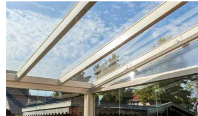
VERANDA WITH GLAZED ROOF
